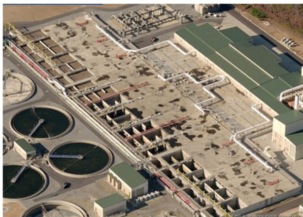
F. Wayne Hill WRC Biological Treatment Basins
