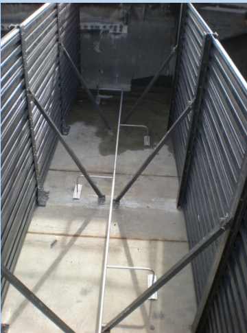
Mixing Header with Nozzles
