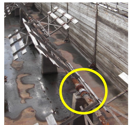
Corroded Mechanical Flocculator
