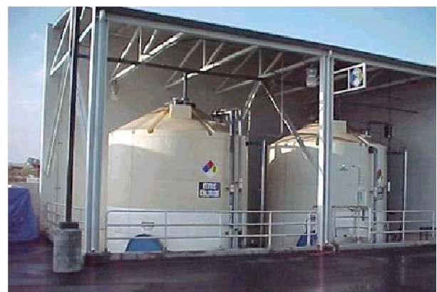
Chemical Feed Storage Tanks
