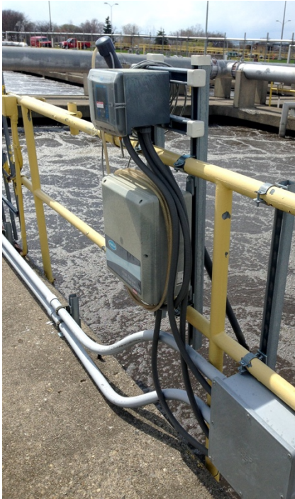
ORP Values in the Anaerobic Selector Zones being mixed with BioMix are typically less than -400 mV.
