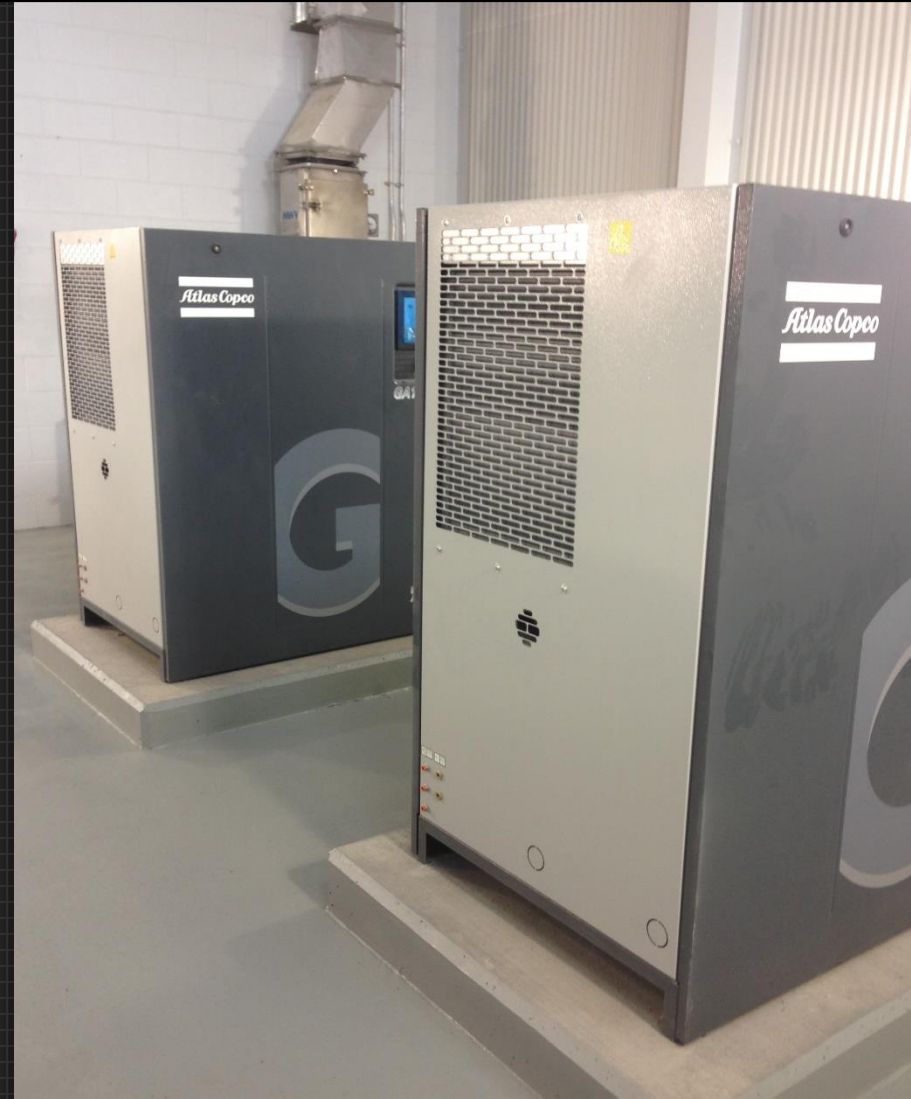
Duty and Standby Compressor
