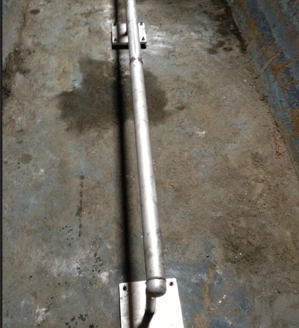
Nozzle Header Installation
