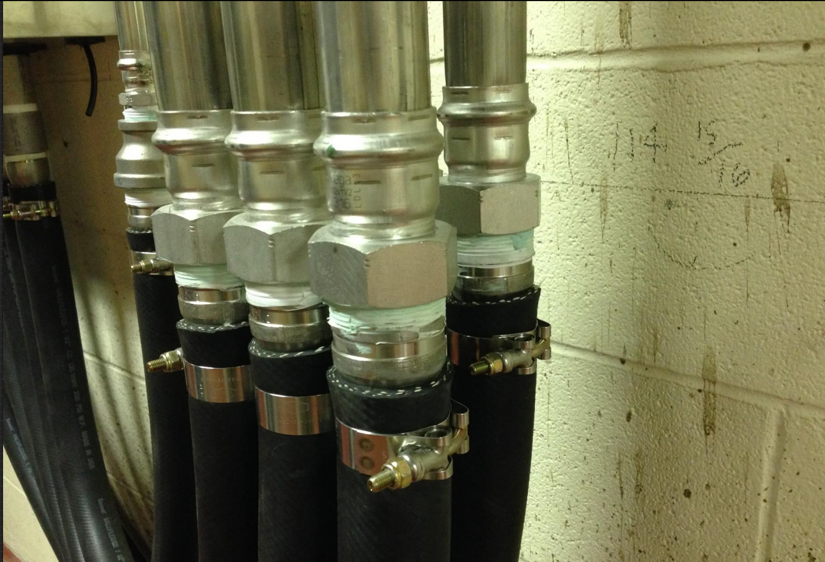
Header Supply Piping is connected to the VCP by Industrial Hose
