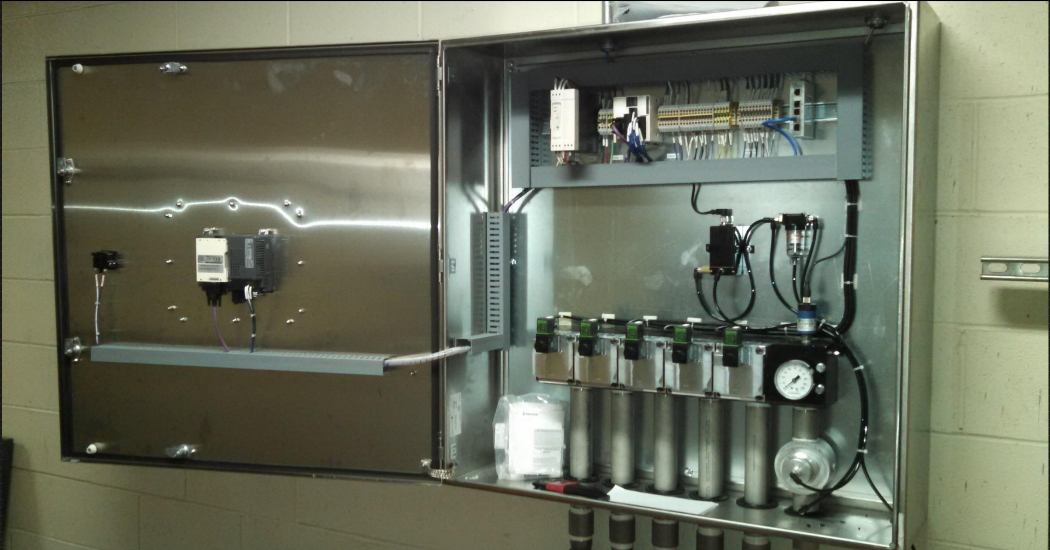
Open Valve Control Panel
