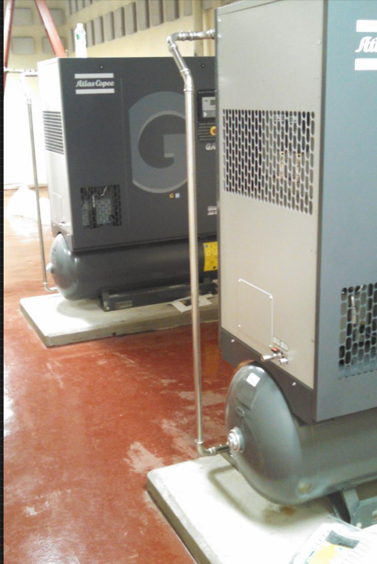
Duty and Standby Air Compressors
