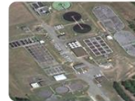
Butner, NC SGWASA WWTP: 6.0 MGD
