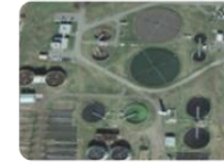
Russellville, AR City Corporation PCWTP: 6.5 MGD
