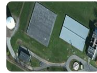
Philadelphia, PA Southwest WPCP: 200 MGD
