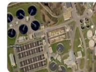
Providence, RI Bucklin Point WWTP: 116 MGD
