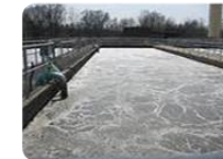
Chambersburg, PA FCGA WWTP: 4.0 MGD
