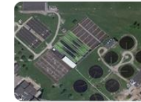
Warren, MI Warren WWTP: 36 MGD
