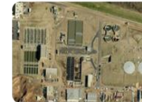
Little Rock, AR Fourche Creek, WWTP: 16 MGD
