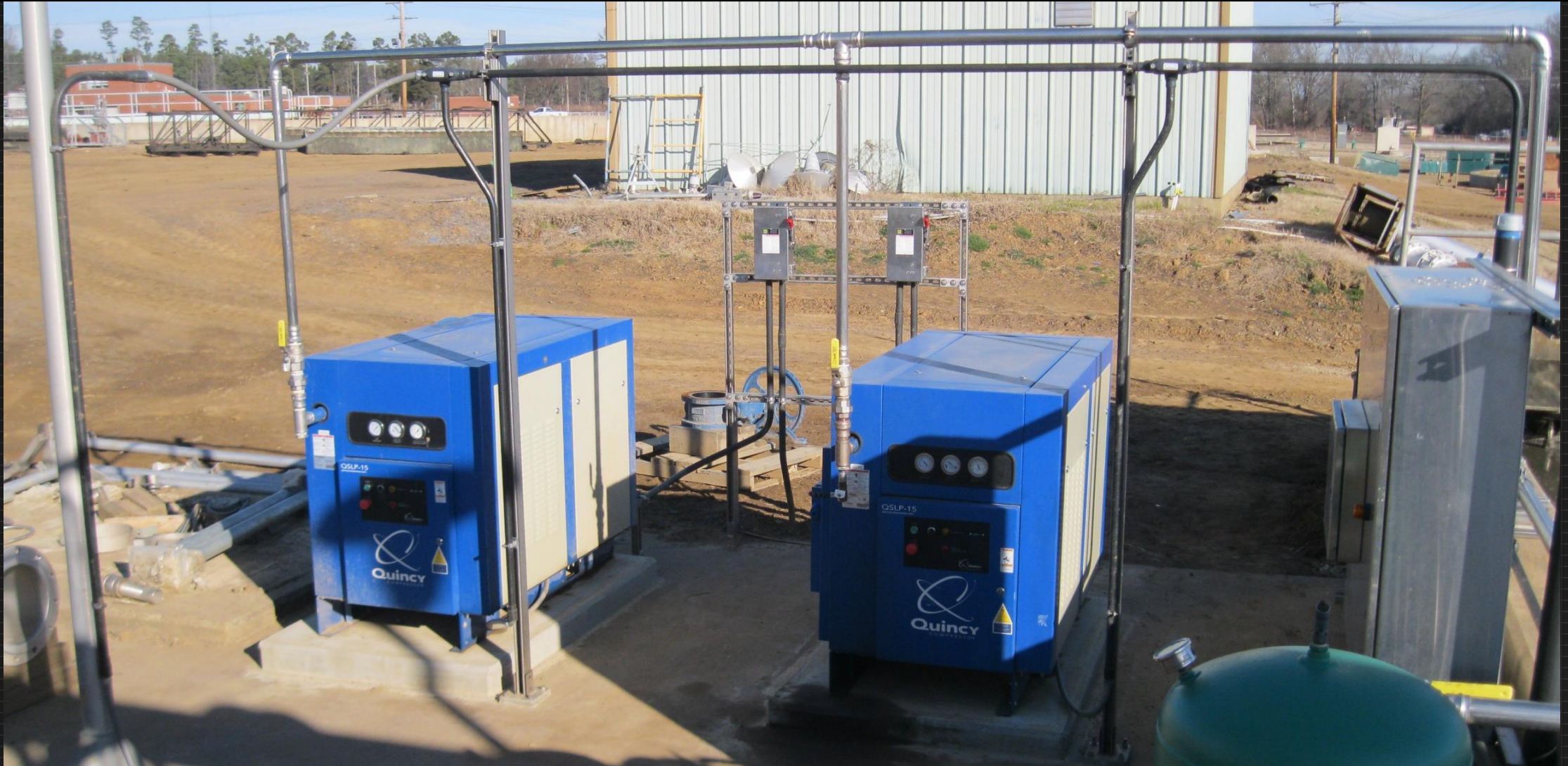
Duty and Standby Compressor
