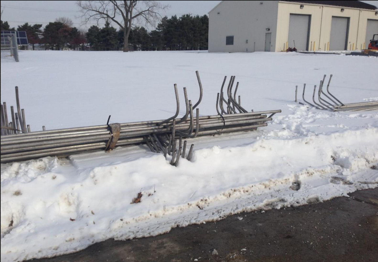
Nozzle Headers Pre-Installation
