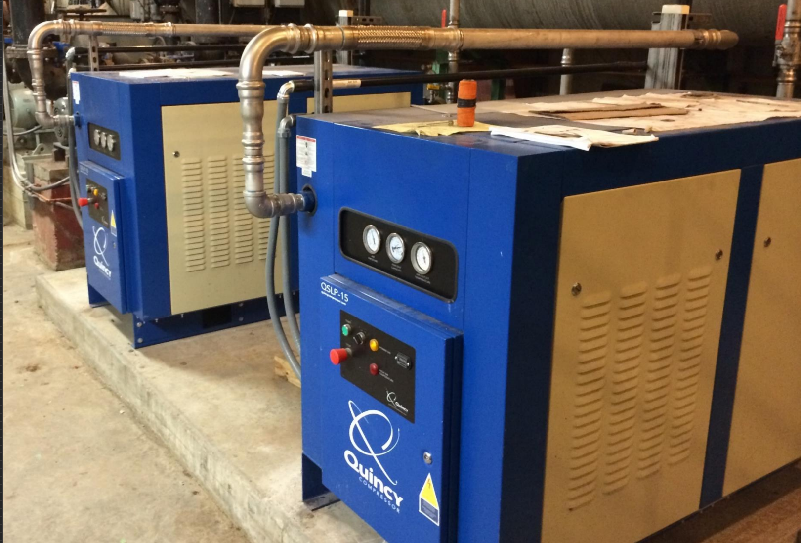
Duty and Stand-by Air Compressors
