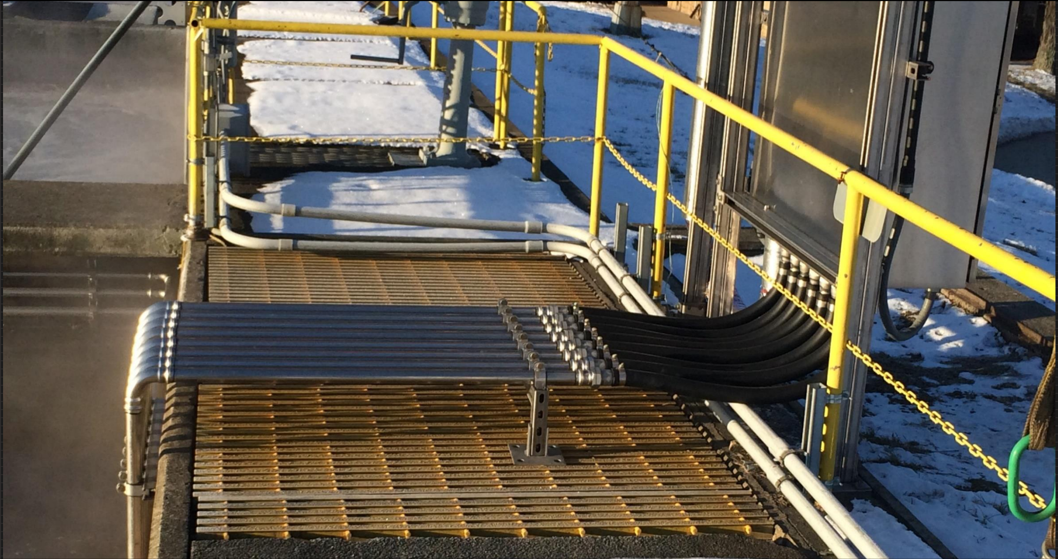
Header Supply Piping from VCP
