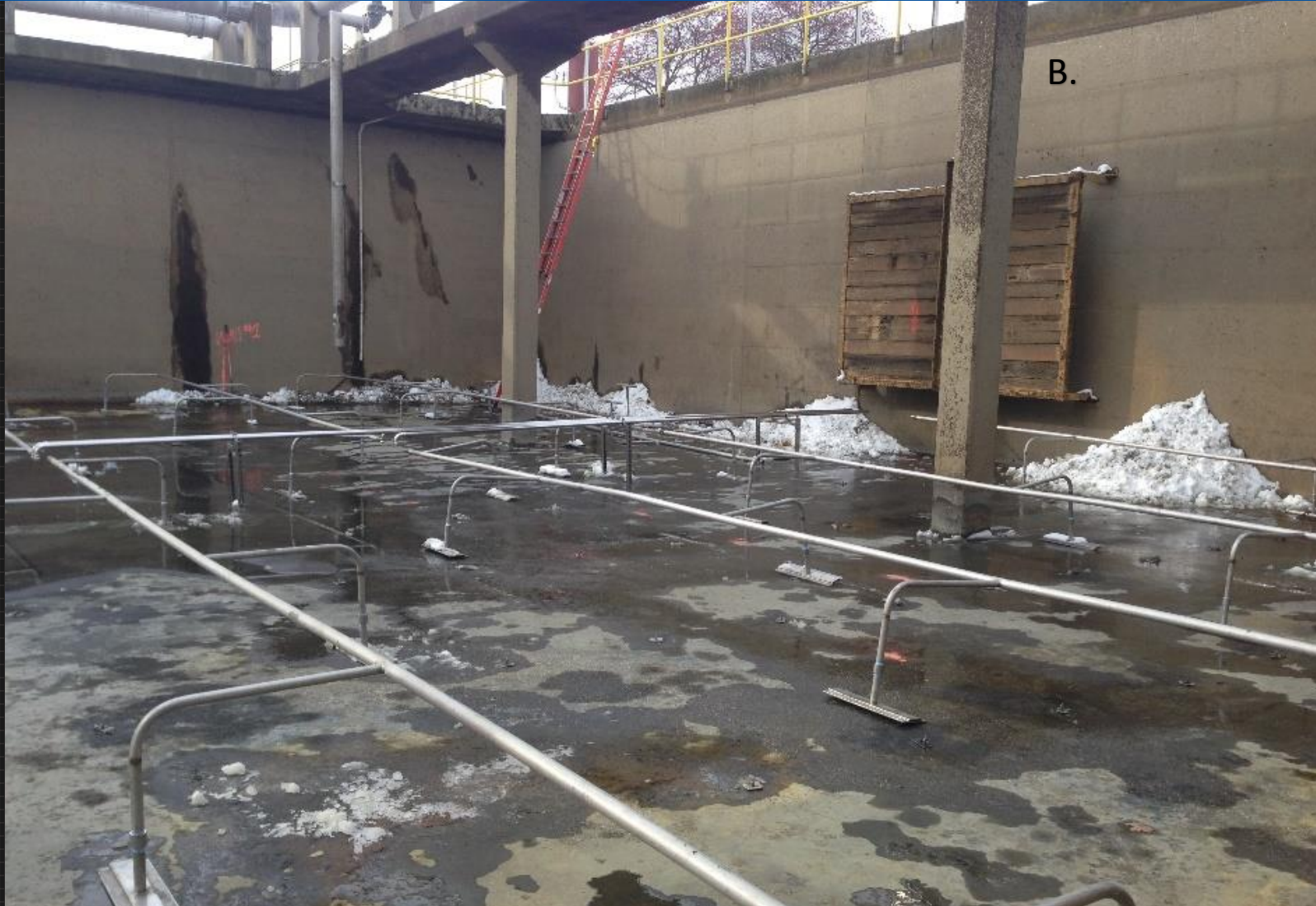
Nozzle Header Installation
