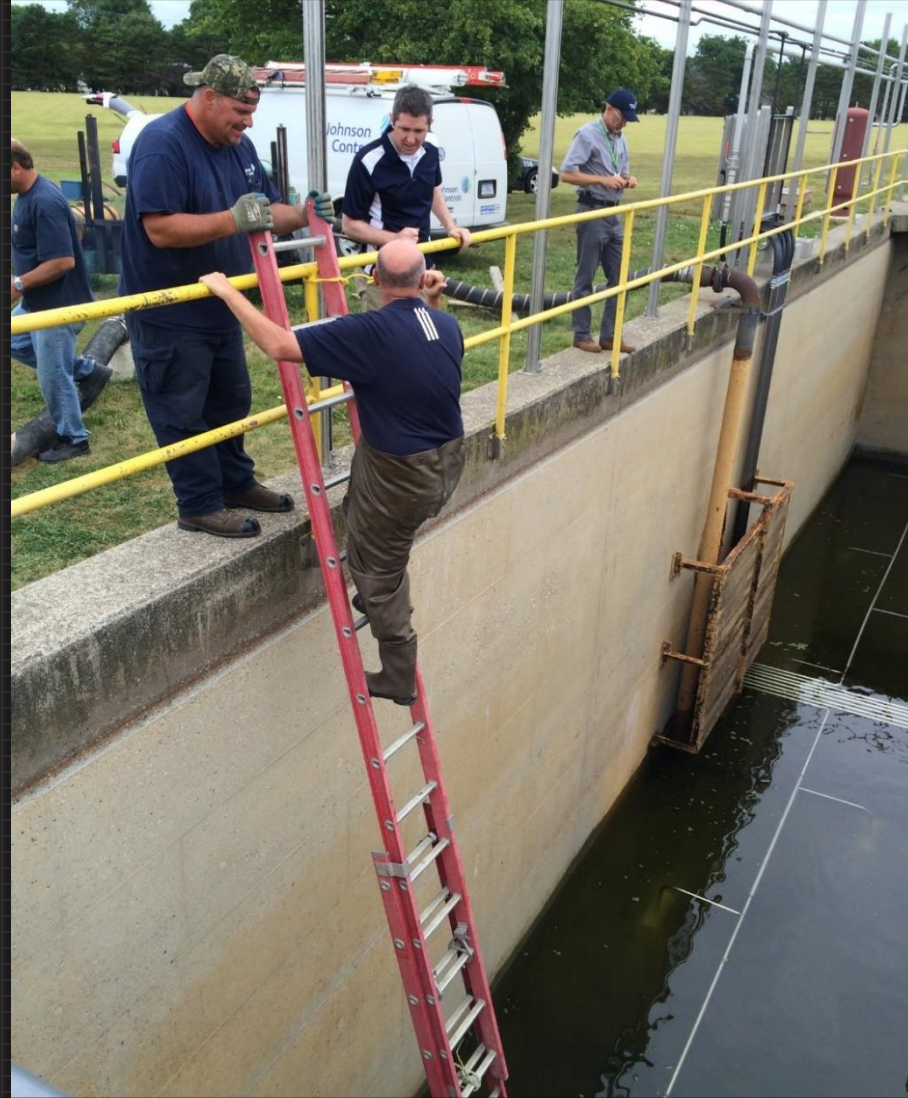
BioMix™ Piping Inspection
