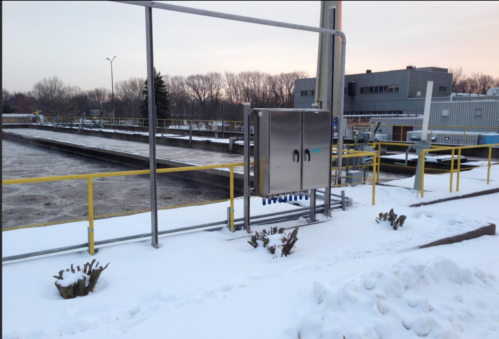
Valve Control Panel (VCP)
