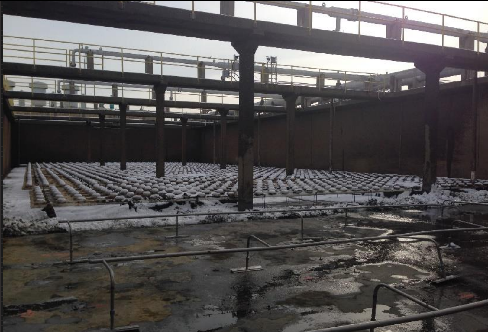
Nozzle Header Installation
