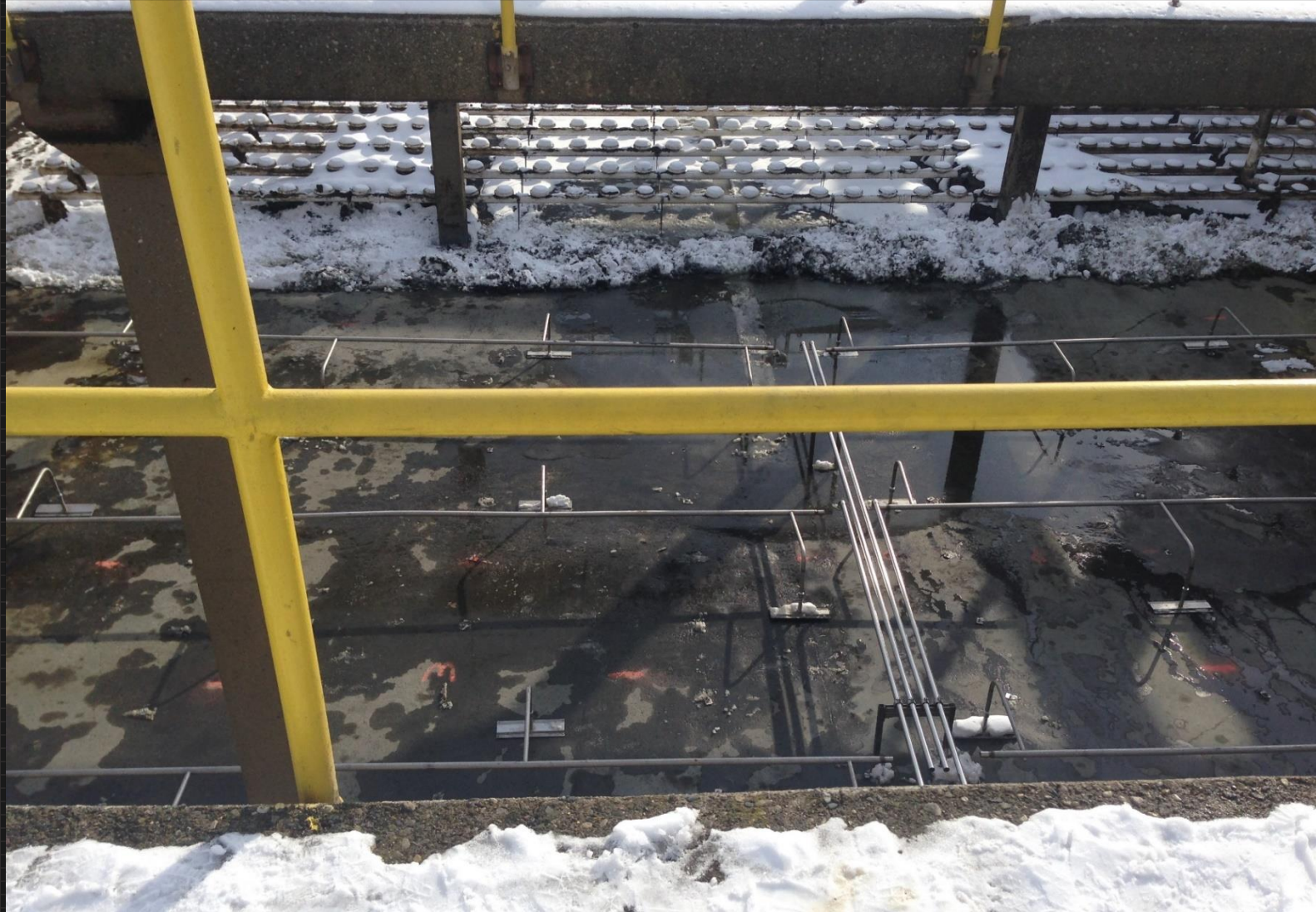
Nozzle Header Installation
