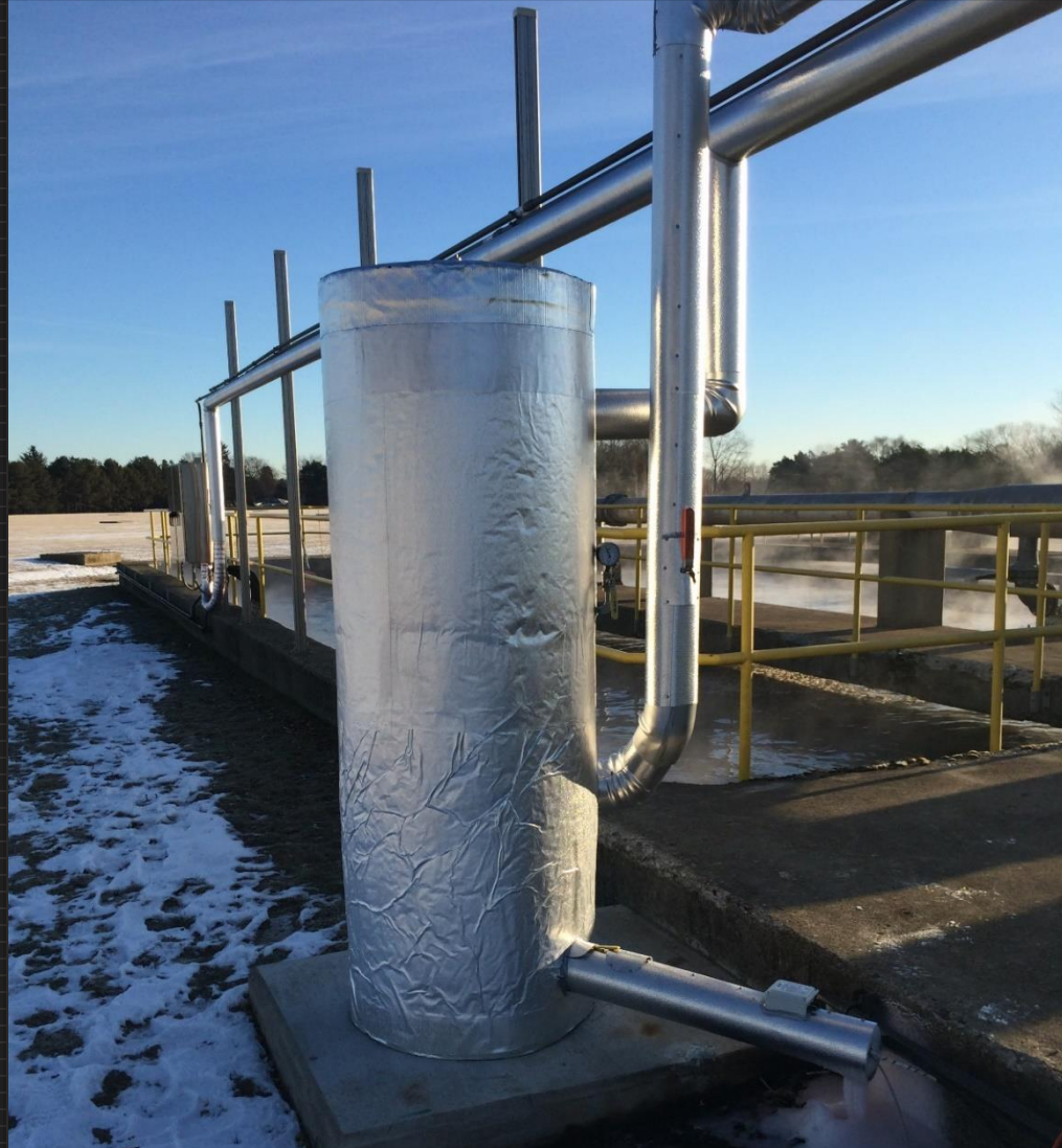
Insulated Air Receiver Tank
