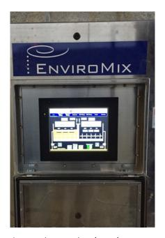
Automatic operation through instrumentation feedback and intuitive operator interface
