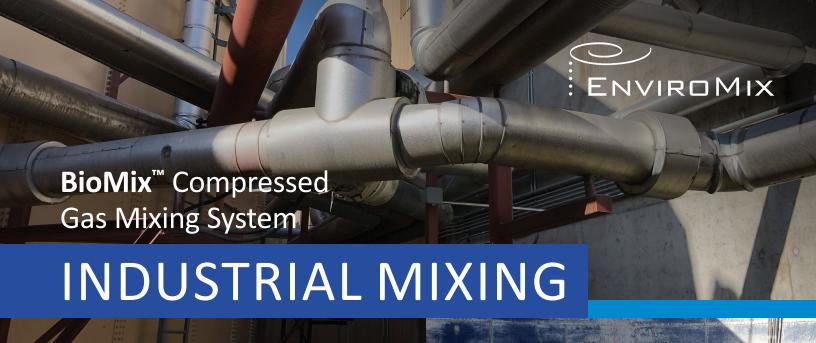
BioMix provides uniform mixing of tank contents by firing programmed, short-duration bursts of compressed air through patented, engineered nozzles located near the tank floor. The mixing parameters may be adjusted to optimize mixing and power utilization, either through operator input or automated process feedback
