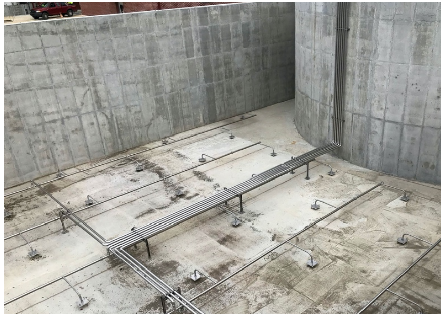
BioMix provides bottom-up, uniformly distributed, energy-efficient mixing.
