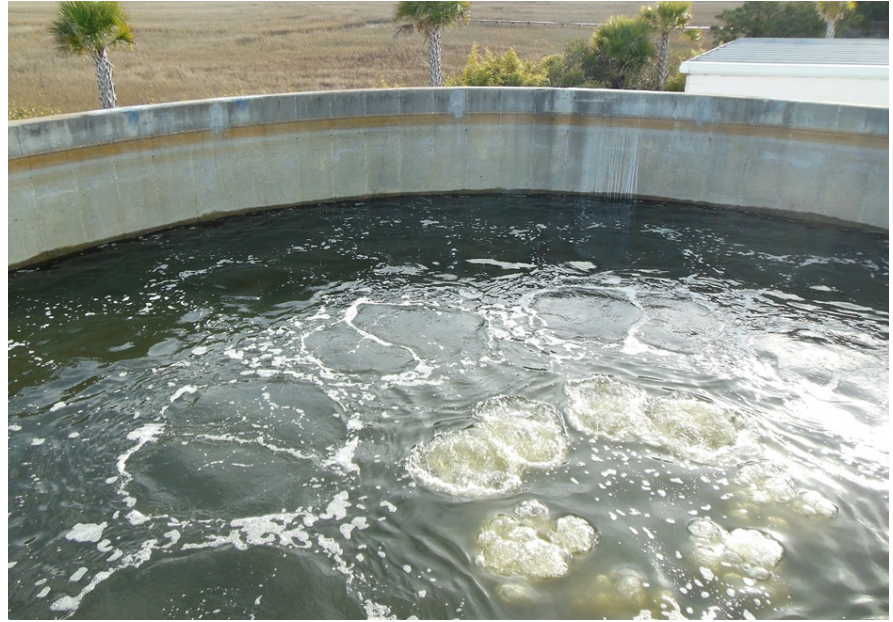
Short duration, sequential bursts of compressed air uniformly mix the tank contents.
