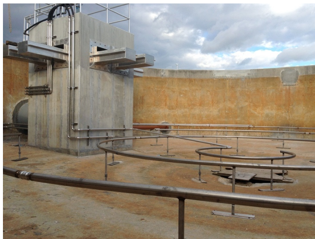
Nozzle headers are custom designed to avoid tank obstructions.
