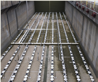
BioCycle-D installation with integrated diffused aeration system and BioMix mixing system.
