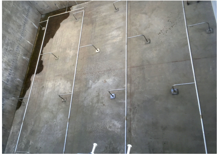
Uniformly spaced nozzles provide effective mixing.
