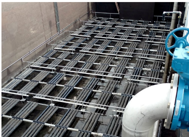
BioMix nozzles and nozzle headers seamlessly integrate with the existing diffused aeration system.
