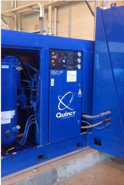
Two 100 HP compressors replaced dozens of mechanical mixers
