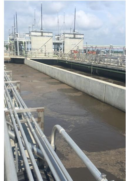
The versatile bioreactors (VBRs) in anoxic operation
