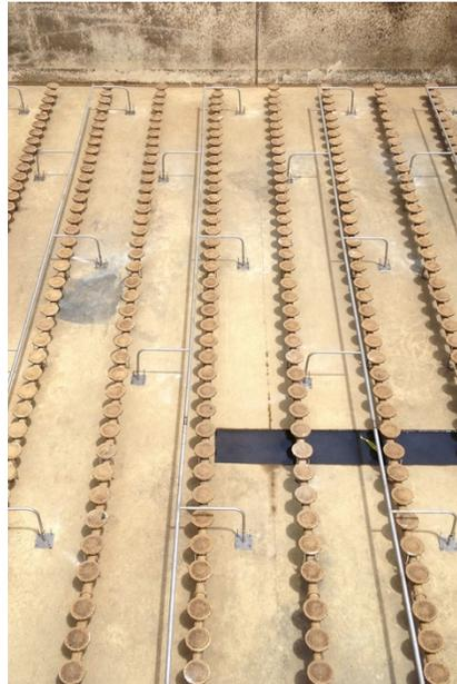
Decoupling aeration from mixing prevents over-aeration
