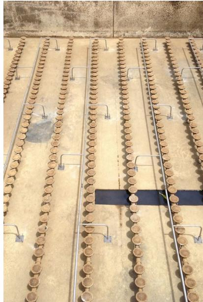
Decoupling aeration from mixing prevents over-aeration
