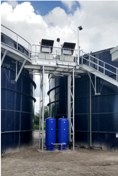
Local control panels distribute the optimal mixing energy.
