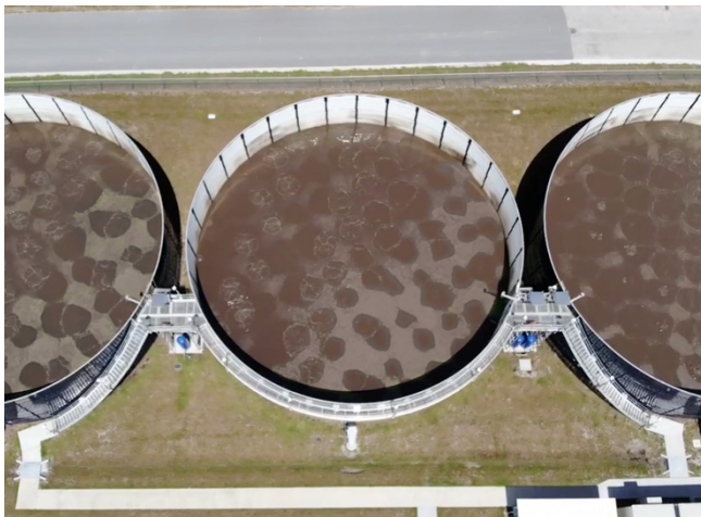
Short duration bursts of compressed air mix an area of the tank 2–3 times per minute.
