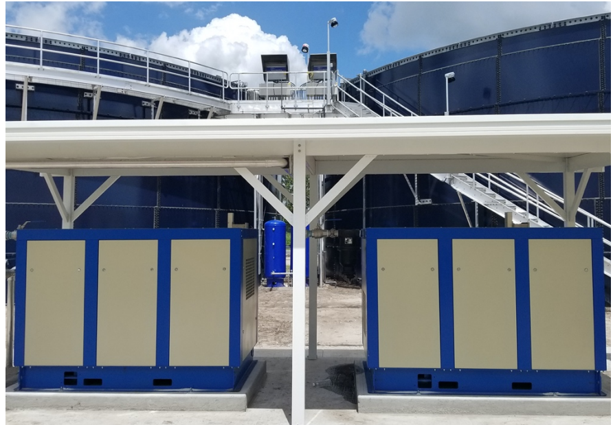
Compressors under a canopy meet the process mixing air demands of the BioMix system for all three equalization tanks.
