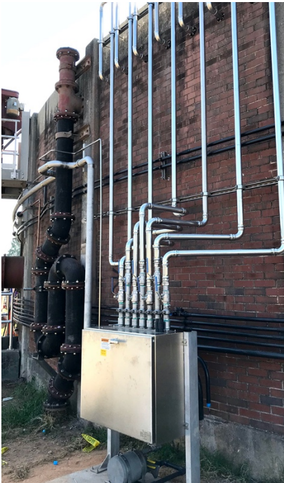
Valve Modules control the firing of compressed digester gas to uniformly mix the digester.
