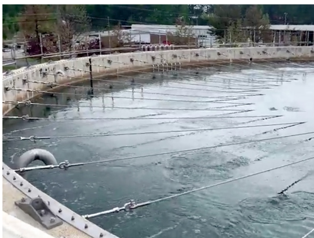
Short duration, intermittent bursts of compressed biogas provide uniform mixing.
