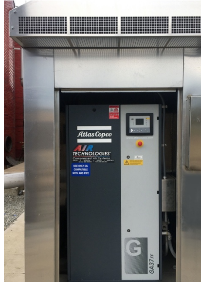
Compressor is housed in an environmental enclosure to eliminate the need to construct a building
