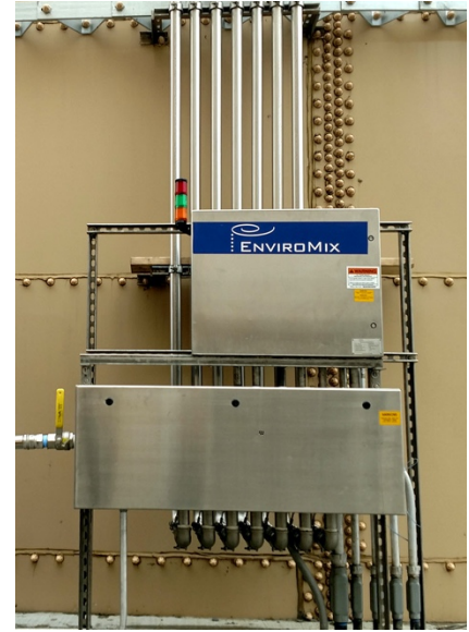
EnviroMix control modules allow for adjustable mixing intensity to match system demands
