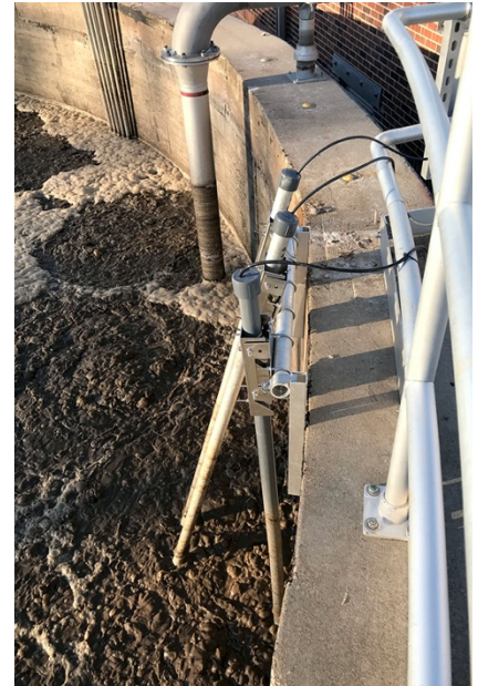
Level, DO, and ORP instrumentation
