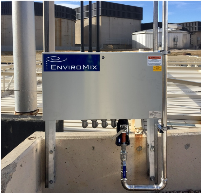
The valve control module enables the optimal mixing regime by controlling air release duration, frequency, and sequence.
