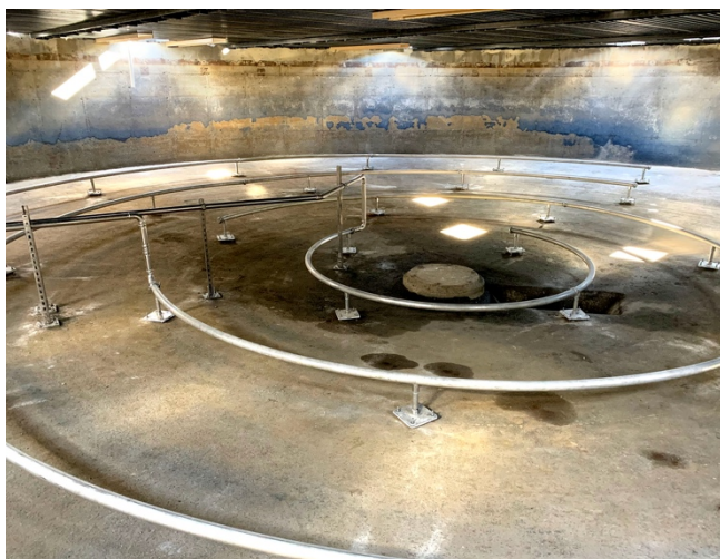
Concentric rings of nozzle headers uniformly mix the basin contents from the bottom up.
