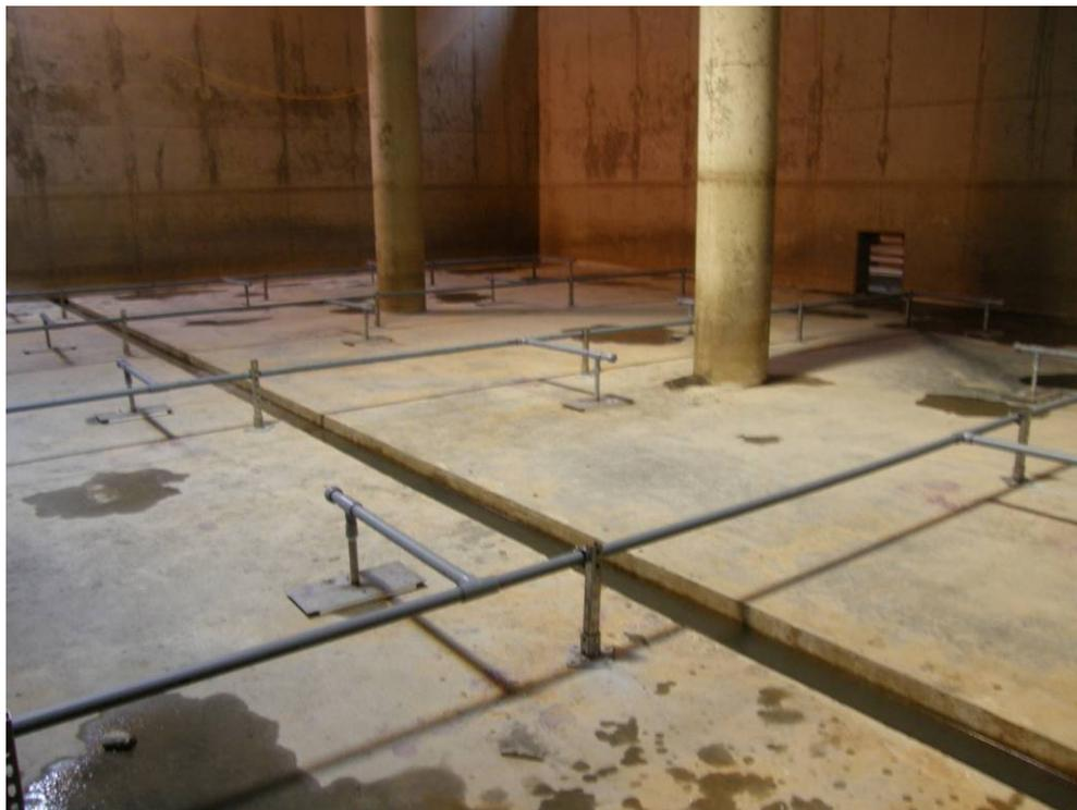
Figure 2c – Bio<sup>M</sup>x and Submersible Mixing Installation, Tank A2 (1' Water Level) Partial View
