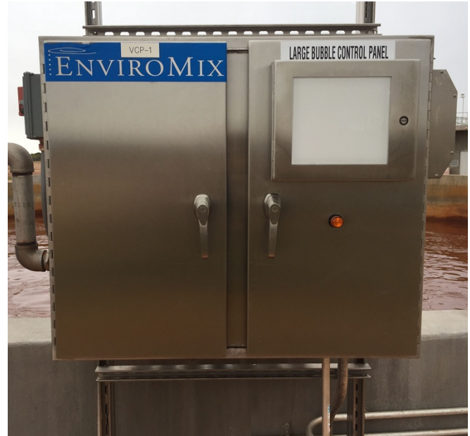
A local valve module provides an operator interface for control of nozzle firing parameters
