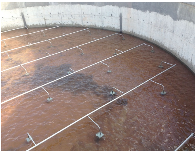
Uniformly distributed nozzles headers provide bottom-up mixing
