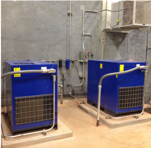
Compressed air is provided by duty and standby compressors
