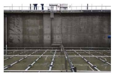
The City of Benton, IL, a 1.65 MGD WWTP, is utilizing a system of decoupled aeration and mixing in its aerobic digesters to realize over \$40,000 in annual energy cost savings. That amounts to roughly 70% savings versus conventional aerobic digestion without any sacrifice to the digestion process – in fact, the process is improved versus diffused aeration alone.
