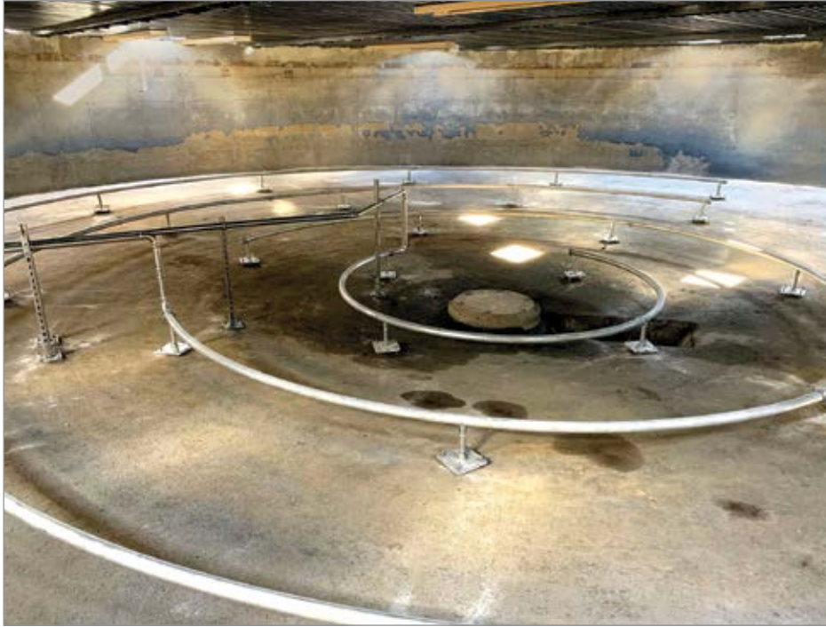
Figure 7: Concentric rings of nozzle headers uniformly mix the basin contents from the bottom up.
