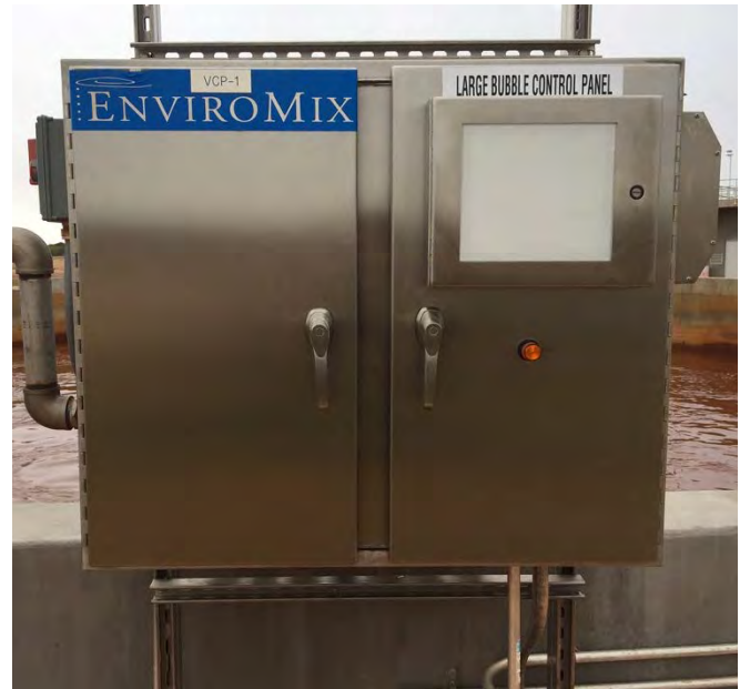
A local valve module provides an operator interface for control of nozzle firing parameters
