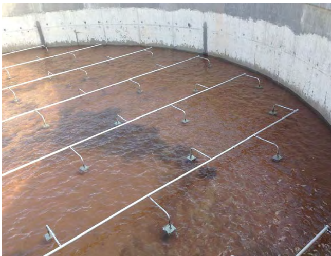
Uniformly distributed nozzles headers provide bottom-up mixing
