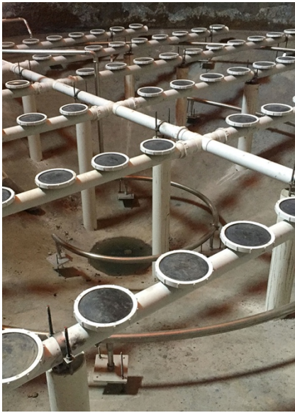
BioMix nozzles in the cone bottom provide bottom-up mixing beneath the aeration grid eliminating dead zones
