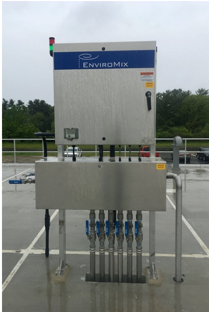
EnviroMix valve modules facilitate adjustment of the mixing intensity to suit process requirements.
