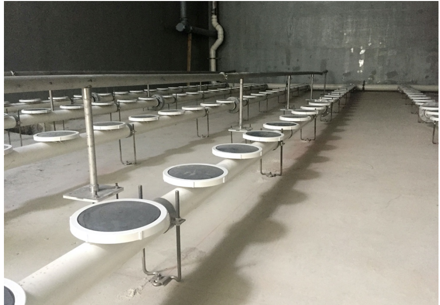
BioMix seamlessly integrates with the fine bubble aeration system within both the swing zones and the aerated sludge holding tanks.
