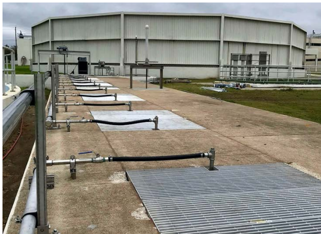
Single drop style nozzle headers uniformly mix the RAS channel
