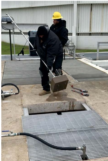
Drop-in nozzle headers uniquely designed for wet installation in an active channel
