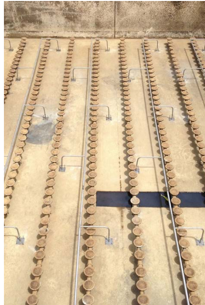
Decoupling aeration from mixing prevents over-aeration
