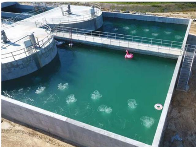
*BioMix Compressed Gas Mixing System operating during startup of anoxic selectors.*
