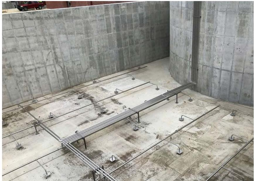
*BioMix provides bottom-up, uniformly distributed, energy-efficient mixing.*
