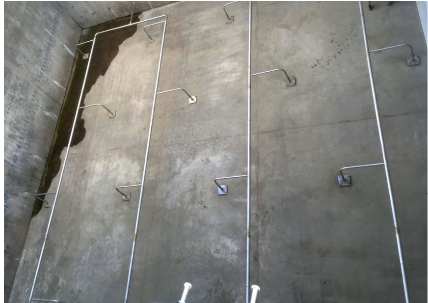
Uniformly spaced nozzles provide effective mixing.
