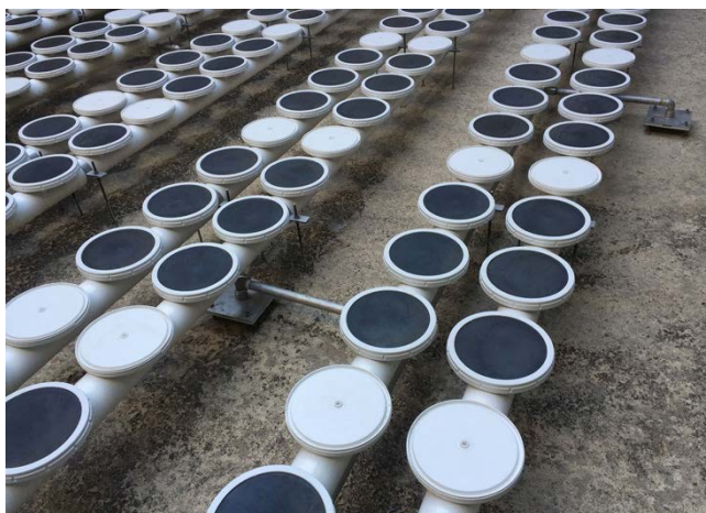
Nozzles seamlessly integrated with diffused aeration
