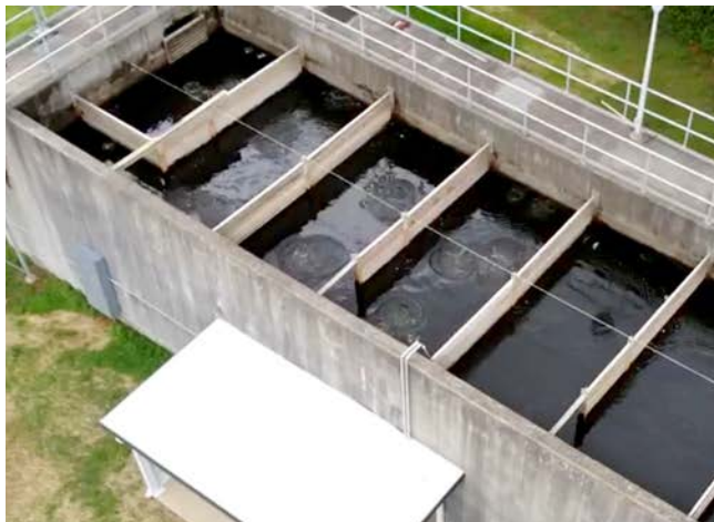
AquaBlend provides efficient and effective mixing in the PAC contactor
