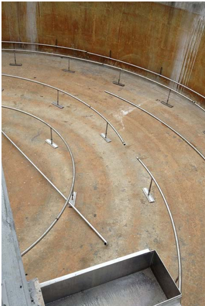
Concentric rings of nozzle headers: Nozzles follow the slope of the tank floor.
