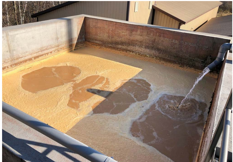
BioMix replaced inefficient jet mixing in the anaerobic selector reducing power use by more than 50%.
