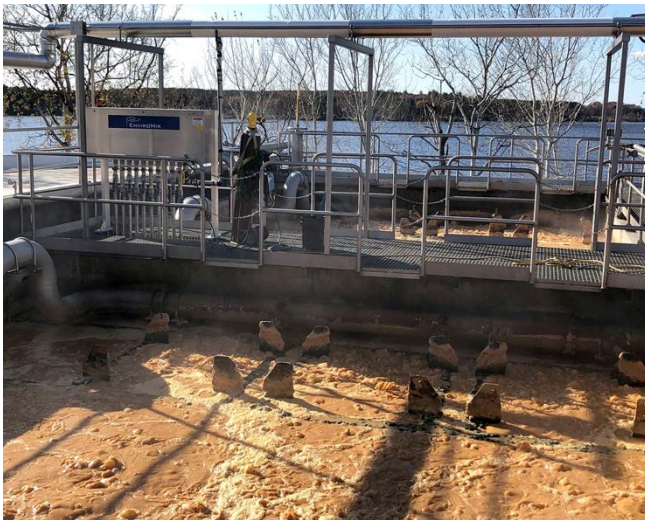
Decoupling aeration from mixing in the MBR basins prevents over-aeration and eliminates solids deposition in the basins.
