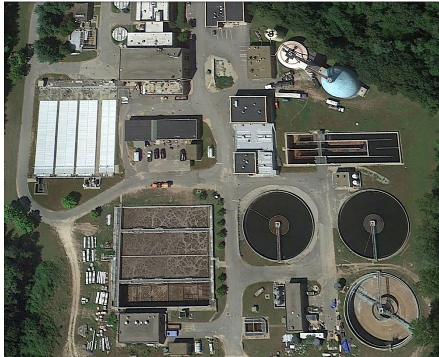
Nashua Wastewater Treatment Facility
