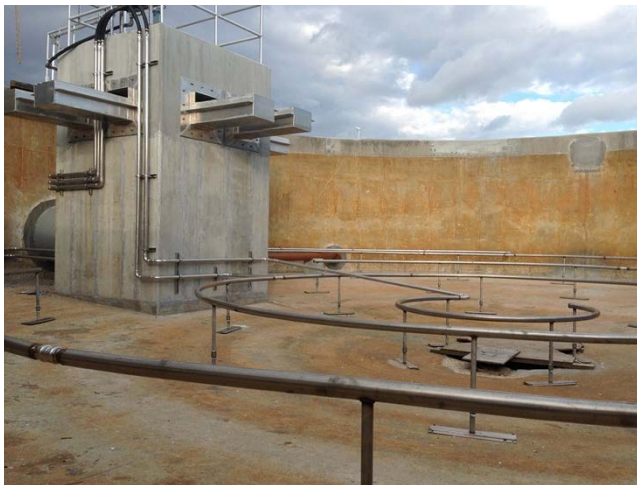
Nozzle headers are custom designed to avoid tank obstructions.
