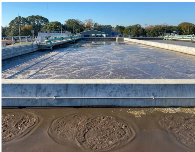
The anoxic zone, mixed by BioMix, provides the optimal conditions for denitrification.
