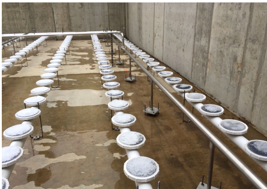
BioMix Compressed Gas Mixing is integrated seamlessly with the fine bubble diffused aeration system to decouple aeration from mixing.
