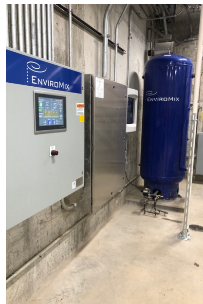
The Master Control Panel controls the BioMix system as well as the blowers through online instrumentation.
