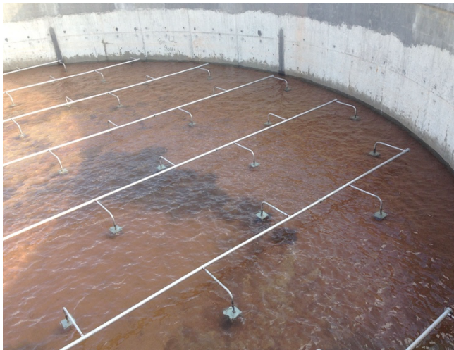
Uniformly distributed nozzles headers provide bottom-up mixing
