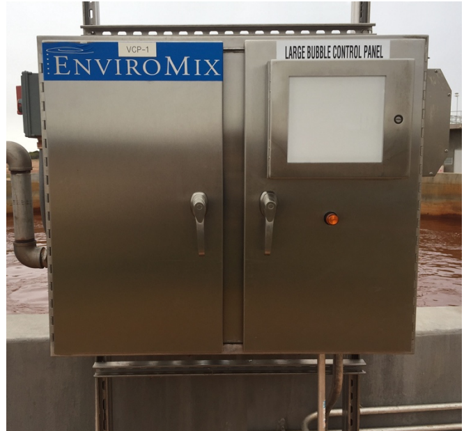
A local valve module provides an operator interface for control of nozzle firing parameters
