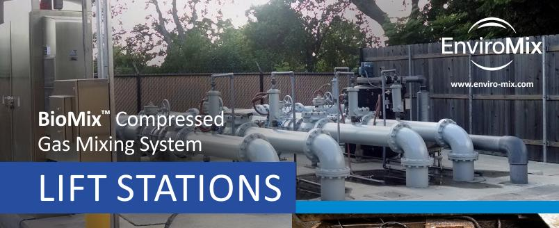
BioMix provides uniform mixing of tank contents by firing programmed, short-duration bursts of compressed air through patented, engineered nozzles located near the bottom of the wet well. The technology is ideal for managing collection of fats, oils and grease (FOG), and keeping a homogenous mixture flowing through the wastewater collection system with minimal inspection and maintenance.
