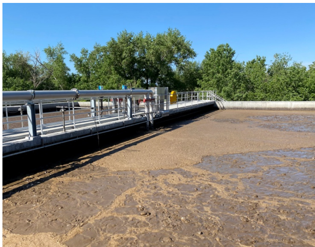
BioCycle-D's alternating aerobic and anoxic cycles maximize VS destruction and improve sludge dewatering.
