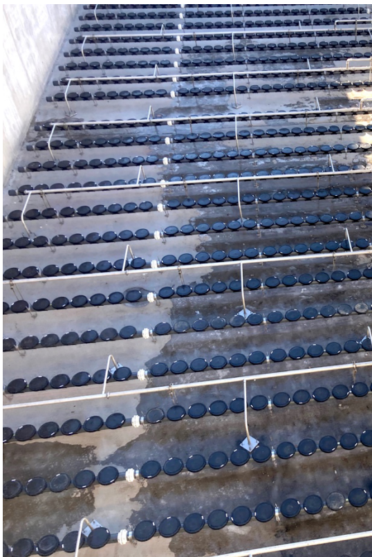
Decoupled fine bubble diffused aeration delivers oxygen and the BioMix Compressed Gas Mixing System provides efficient mixing.
