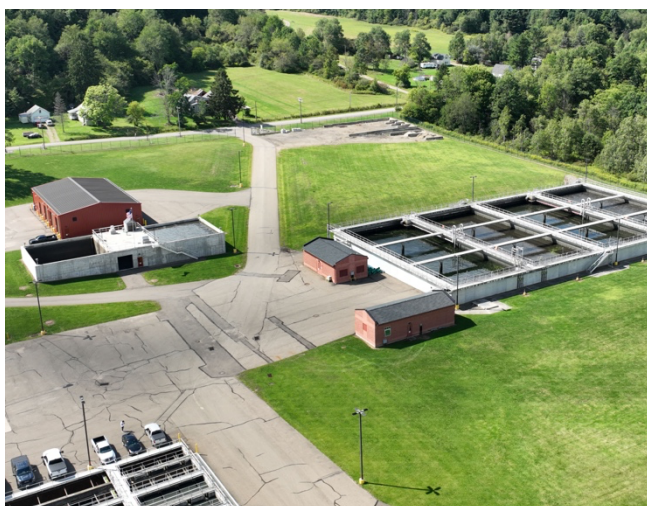
Bradford's wastewater treatment plant
