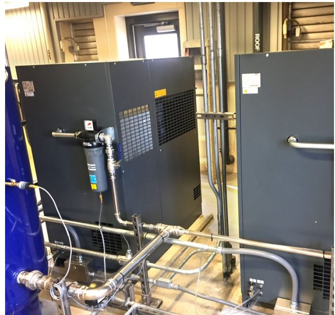
Low maintenance compressor system matches mixing air demand with duty and standby configuration.
