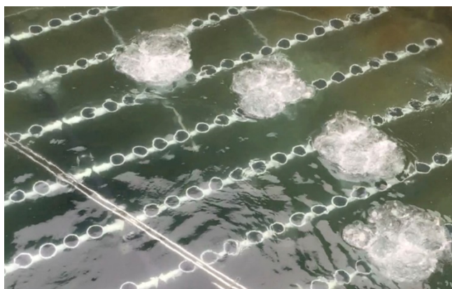
Decoupled aeration from mixing
