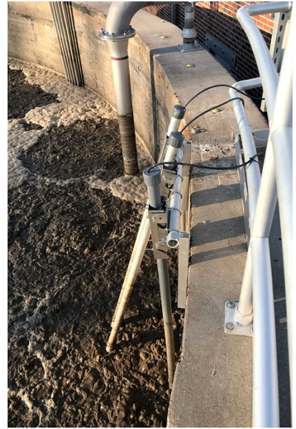
Level, DO, and ORP instrumentation
