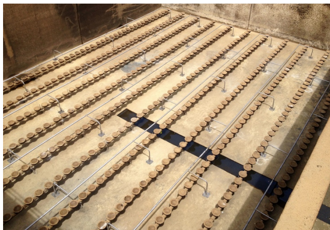
Aeration satisfies oxygen demand while BioMix compressed gas mixing maintains mixed liquor suspension
