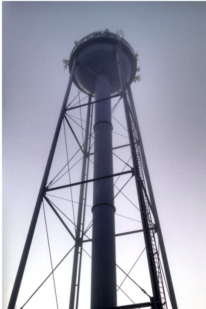
The elevated water storage tank at the Montana Law Enforcement Academy in Helena, MT.
