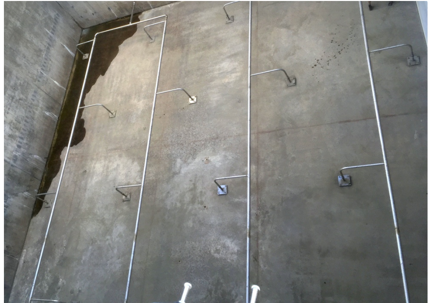
Uniformly spaced nozzles provide effective mixing.
