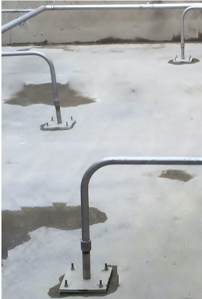
Nozzles mounted at the tank floor maximize bottom-up mixing regime.
